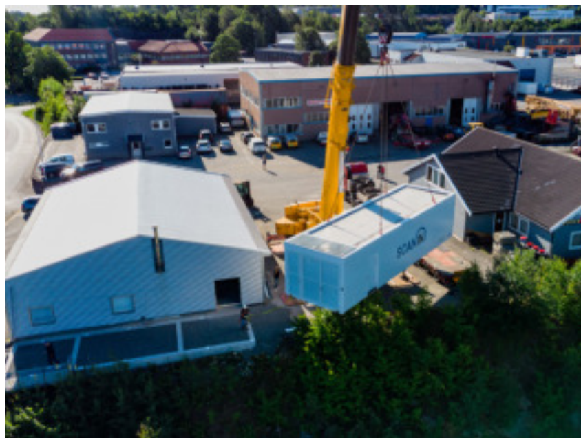
The installation of Canon's first relocatable MRI in Arendal in southern Norway.
