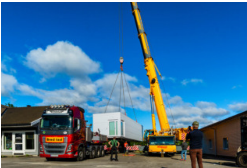
The installation of Canon’s first relocatable MRI in Arendal in southern Norway.
